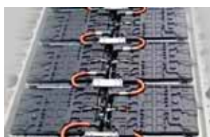
Battery charge/discharge test
